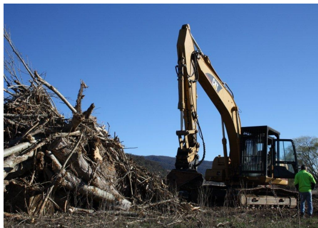
Excavator piling cut willow at Bumbalong Homestead. Photo: Helen Shimitris
